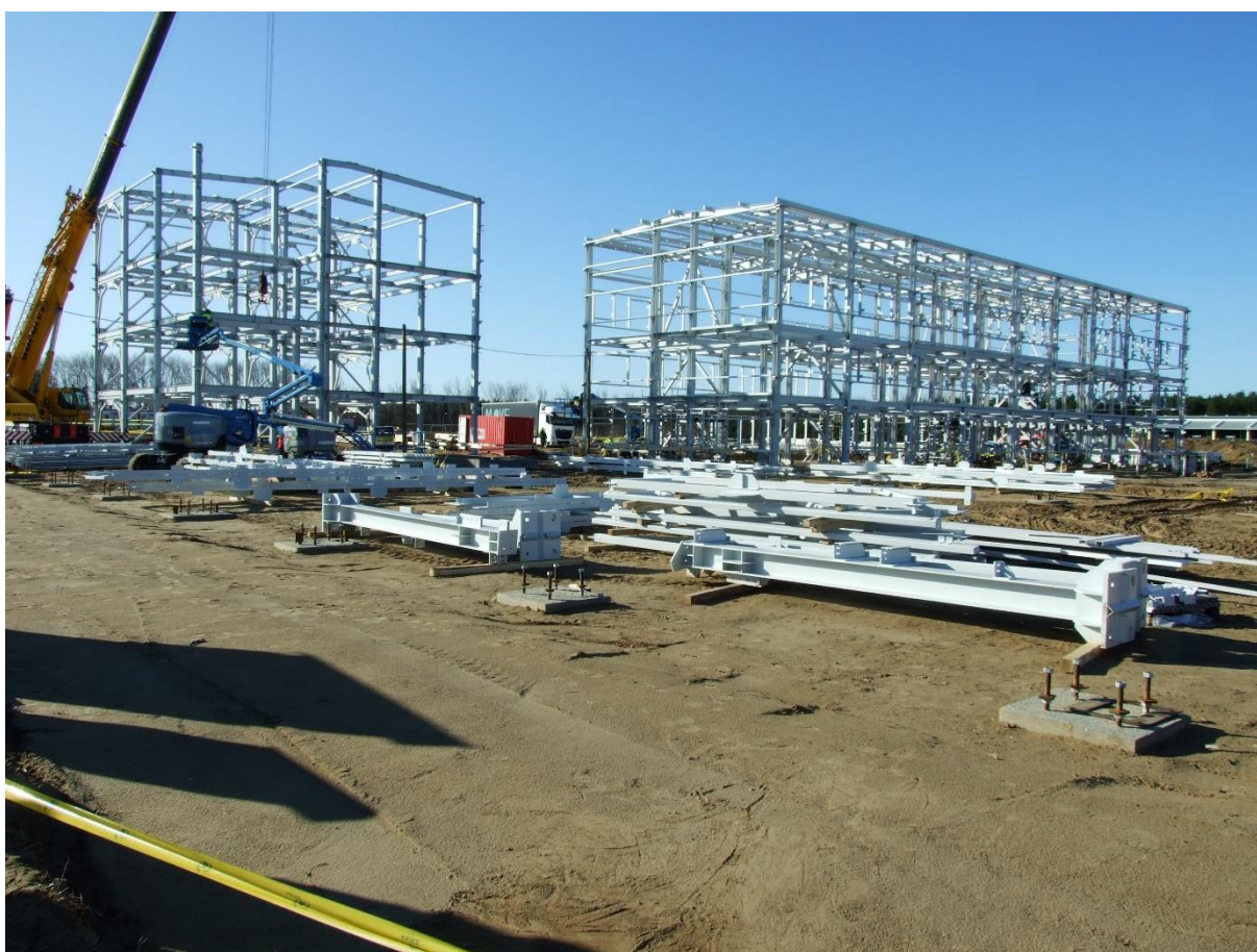
Progress of the buildings of the construction erection base
